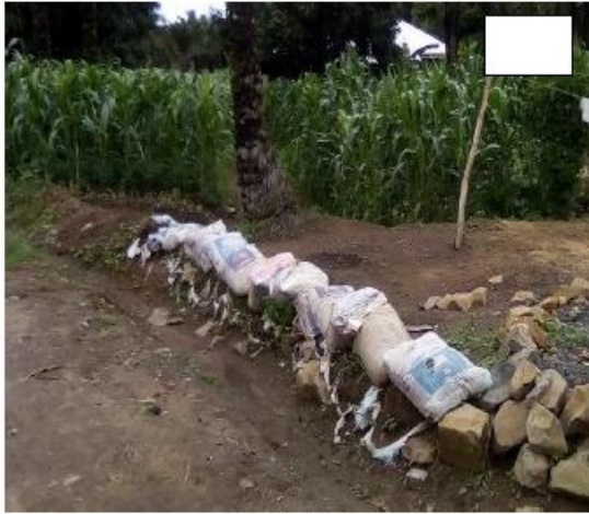
Figure 13a and 13b: Sand Bags Constructed in Some Parts of the Division
