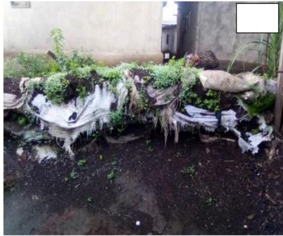
Figure 13a and 13b: Sand Bags Constructed in Some Parts of the Division
