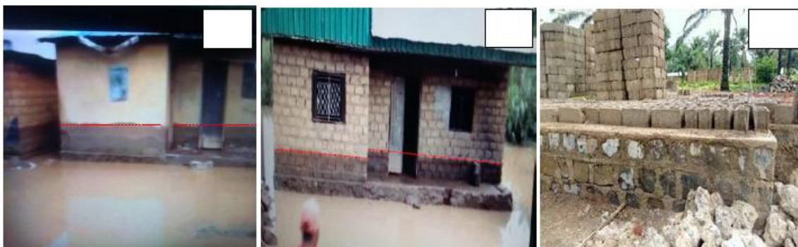
Figure 9: Designed Heights of Some Foundations in the Flood Prone Zones of Ngoketunjia
