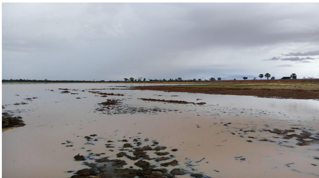
Figure2. The Daberam dam heavily silted with little water contained in it.
