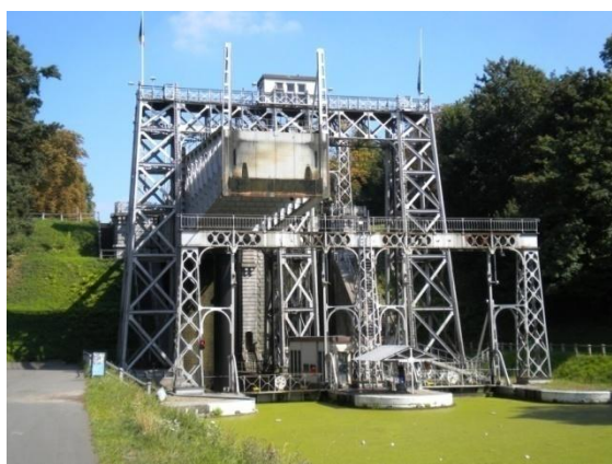
Figure 1. Hydraulic boat-lift of the historic Canal du Centre, Belgium. World Heritage List (Author: Carlos J. Pardo)
