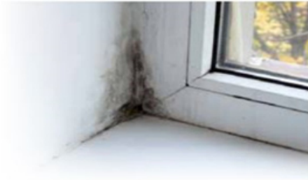
Mold spores: Is part of a fungus. They can be found in a lot of homes. Mold chooses to grow in humid places like bathrooms or kitchens.
