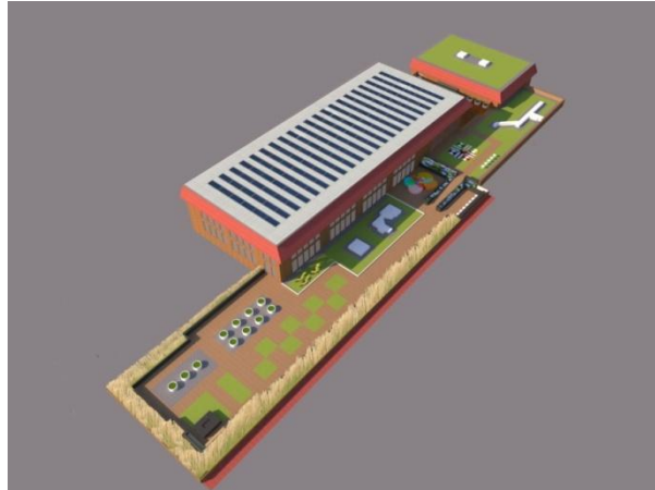
Figure5. Birdseye view of a semi-intensive green roof (treatment 4). (Copyright © 2019 Wing Chi Vincy Tam all right reserved used by permission).
