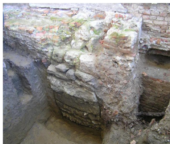
Figure3. The Foundation of the Brick, the Stone Foundation and Closed the Entrance to the Crypt
