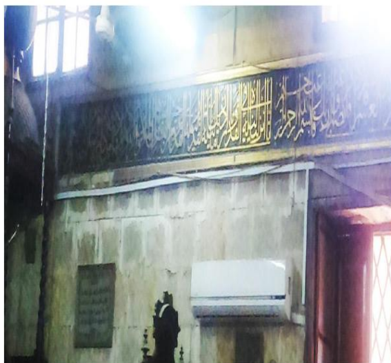
Figure17. Top and Bottom (Zoom in) pictures are showing the formation of "Efflorescence" around plastic conduits extended over the walls of the
