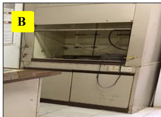
Figure 1(A). A very old bench with some serious damages. (B) An out dated fume hood with rusty cabinets.
