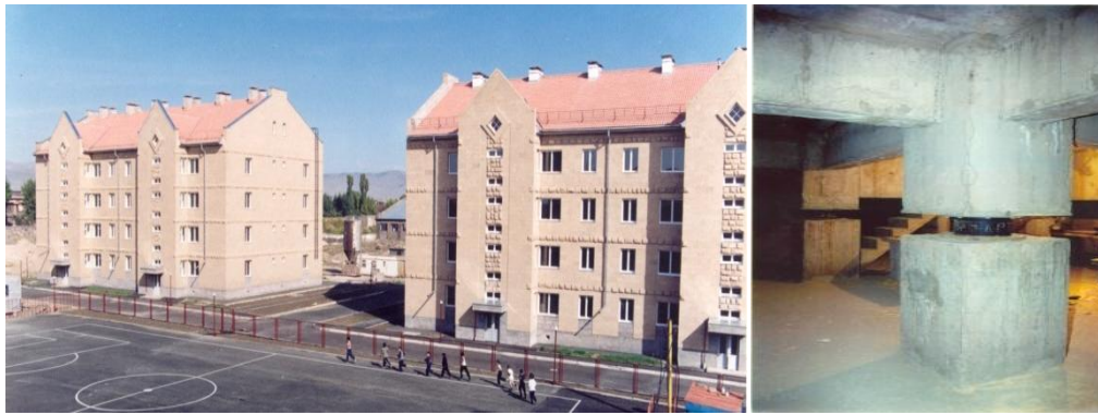
Figure4. Two 4-story apartment buildings in the Huntsman Village of the city of Gyumri and fragment of its isolation system
