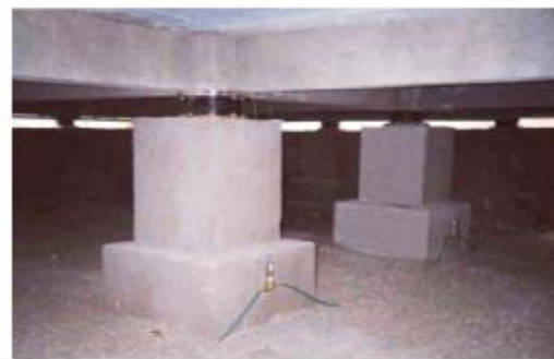
Figure3. 4-story apartment building in the city of Spitak and fragment of its isolation system
