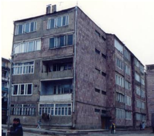
Figure17. First existing 5-story stone apartment building in Armenia retrofitted by base isolation (technology invented by the author) in the city of Vanadzor and fragments of its isolation system. This building was retrofitted for the first time in the world without interruption of its use, so, that during retrofitting works people were not moved out of the building (Melkumyan, 1994, 2002, 2006b, 2009)
