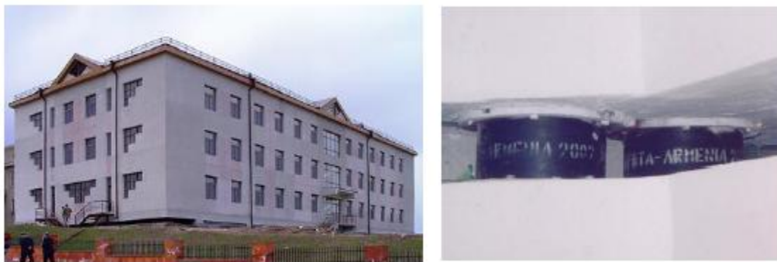
Figure5. 3-story clinic building in the city of Stepanakert and fragment of its isolation system
