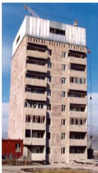
Figure18. 9-story existing apartment building retrofitted by roof isolation (invented by the author method of Additional Isolated Upper Floor - AIUF) in the city of Vanadzor, its design model and fragment of its isolation system. This building was retrofitted in parallel with reconstruction works going on in all floors (Melkumyan, 2007, 2009, 2011)
