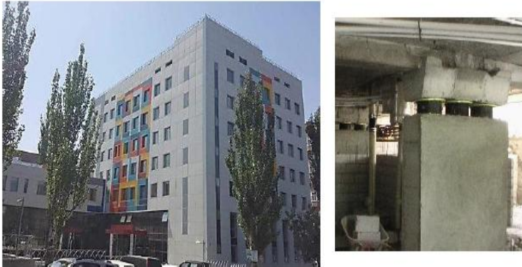
Figure 21. 9-story existing Hematology Center Hospital building retrofitted by base isolation in the city of Yerevan and fragment of its isolation system. This building was retrofitted in parallel with reconstruction works going on in all floors (Melkumyan, 2014d, 2015a, 2019)
