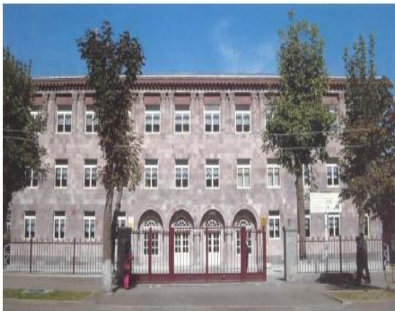
Figure20. 3-story existing school building retrofitted by base isolation in the city of Vanadzor and fragments of its isolation system. At the time of retrofitting the building was 60 years old. This building, which has historical and architectural value, was also retrofitted without interruption of its use (Melkumyan, 2005, 2011, Melkumyan & Hakobyan, 2005)
