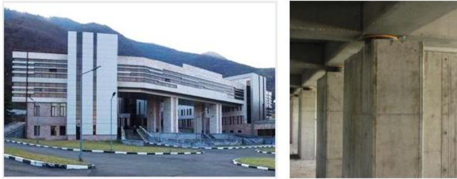
Figure7. 4-story building of medical center in the city of Vanadzor and fragment of its isolation system
