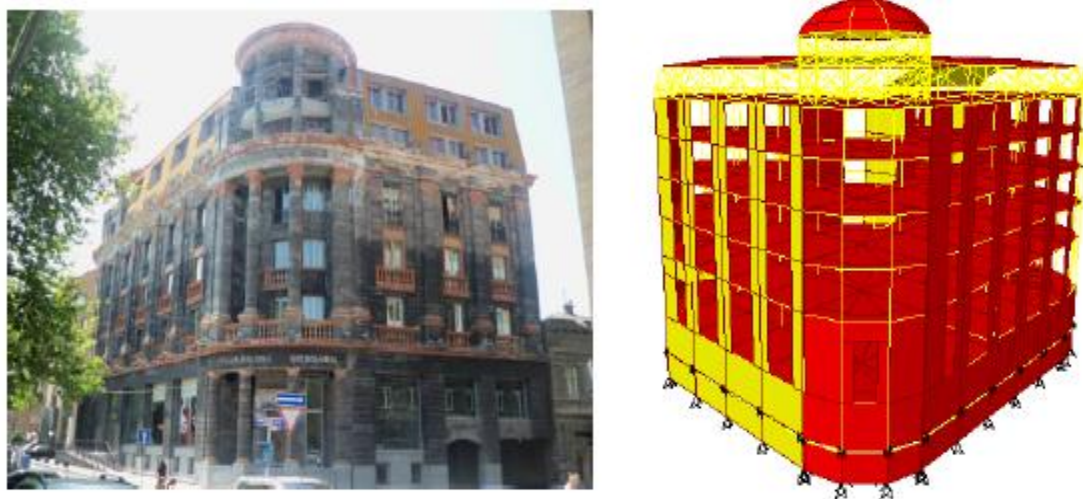
Figure6. 7-story commercial center/hotel building in the city of Yerevan and its design model
