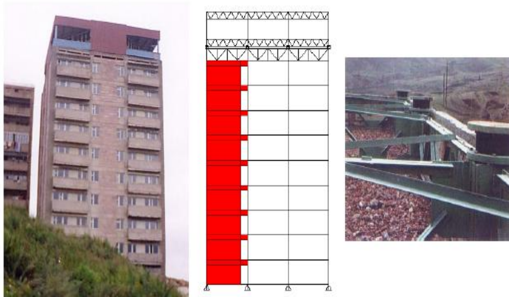
Figure19. 9-story existing apartment building retrofitted by roof isolation (also by the method of AIUF) in the city of Vanadzor, its design model and fragment of its isolation system. This building was also retrofitted in parallel with reconstruction works going on in all floors (Melkumyan, 2007, 2009, 2011)
