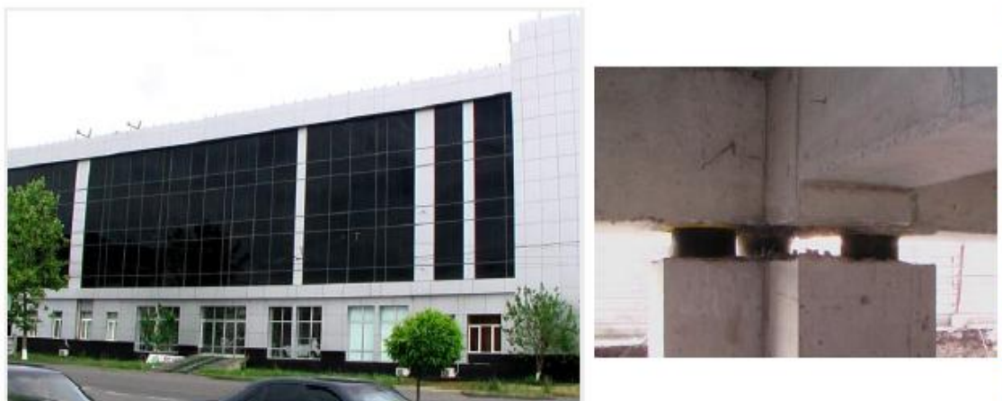
Figure 22. 4-story existing industrial building with R/C bearing frames retrofitted by base isolation in the city of Yerevan and fragment of its isolation system. This building was converted into hotel and was retrofitted in parallel with reconstruction works going on in all floors (Melkumyan, 2014a, 2019)
