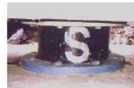
Figure17. First existing 5-story stone apartment building in Armenia retrofitted by base isolation (technology invented by the author) in the city of Vanadzor and fragments of its isolation system. This building was retrofitted for the first time in the world without interruption of its use, so, that during retrofitting works people were not moved out of the building (Melkumyan, 1994, 2002, 2006b, 2009)
