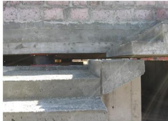
Figure17. Views of the outside double-flight stairs leading from ground level to the first living floor of one of the residential houses; the seismic isolation system, the main gap around the perimeter of the ground floor and the gap in the double-flight stairs
