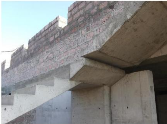
Figure17. Views of the outside double-flight stairs leading from ground level to the first living floor of one of the residential houses; the seismic isolation system, the main gap around the perimeter of the ground floor and the gap in the double-flight stairs
