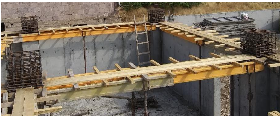
Figure12. View of the reinforcement frames of upper pedestals
