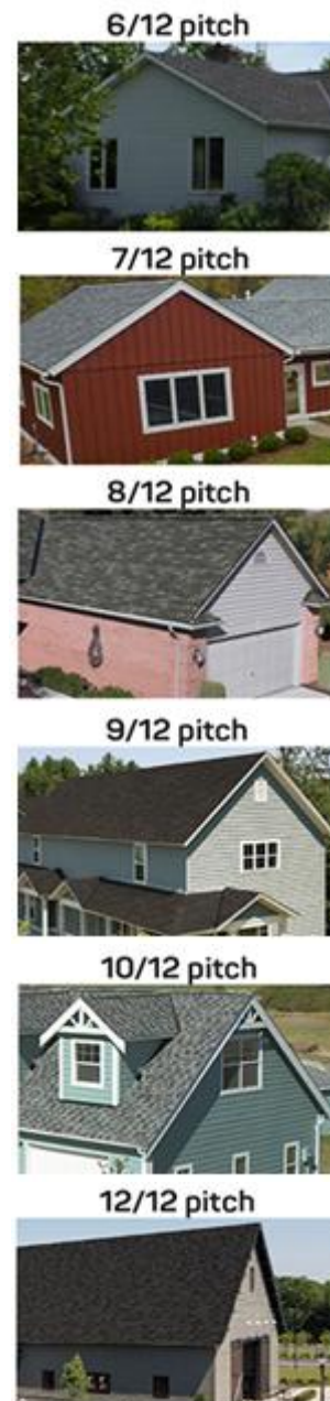
Fig 12. Minimum Slope for an Asphalt Shingle Roof 12
