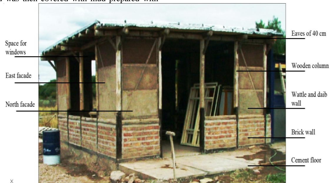
Figure 11. Workshop construction stage.
