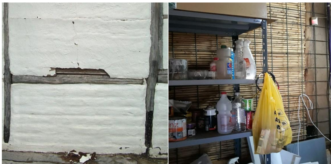
Figure 13. Pathologies in south-facing wattle and daub panels, outside and inside surfaces.
