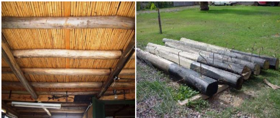
Figure 8. Cane roof and eucalyptus wood columns.
