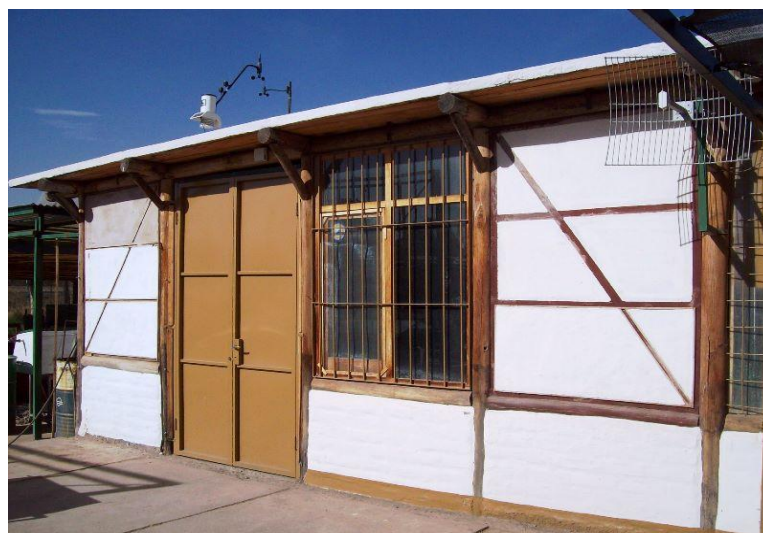
Figure 9. Workshop with finished wattle and daub walls
