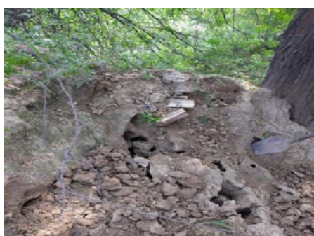
(e). Site of mound for installation
